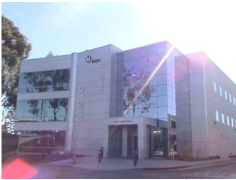
El Monte MTA Division 9 building
